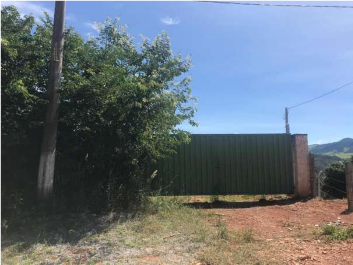
Figura 3 – Entrada Principal do Residencial
